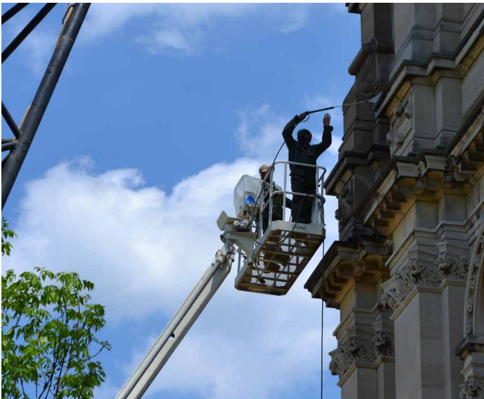
A worker operates the power-washer from the wire-mesh platform.
